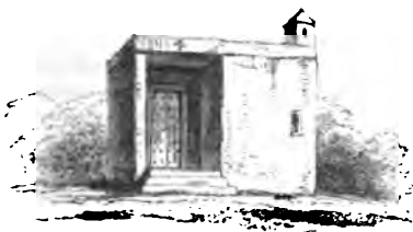
[344.] Hut of Greek peasant, formed of mud embedding sticks and straw. Valley of Xanthus.—Fellows' Lycia.
